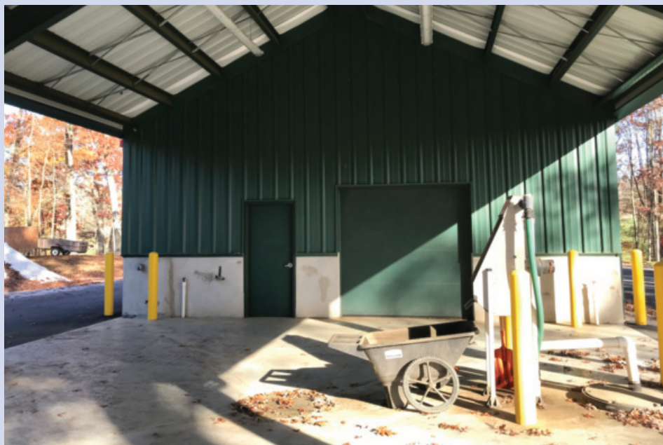
Bedford Golf & Tennis Superintendent Bob Neilsen tackles several BMPs with the club's new pesticide storage/mixing/loading and equipment wash pad building.
